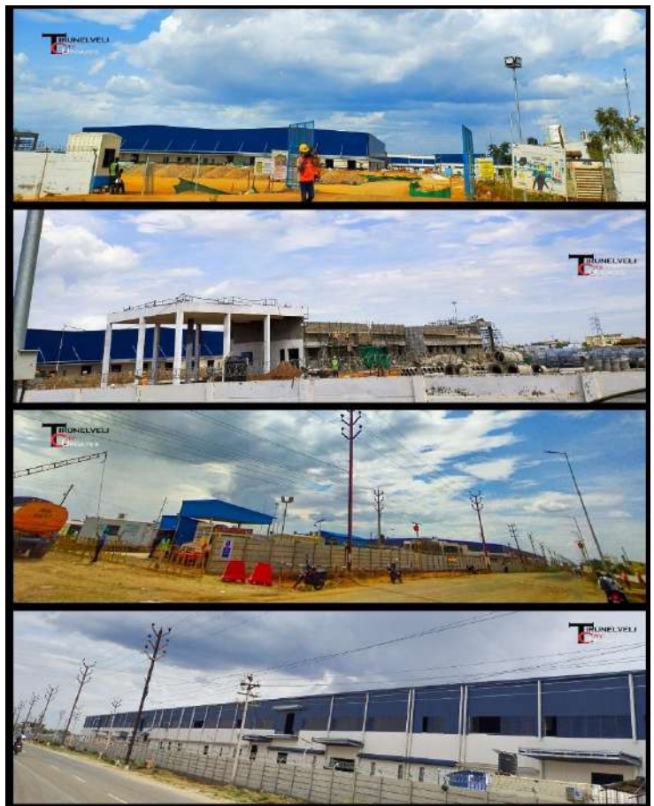
Figure 4.18 TP SOLAR UNDER CONSTRUCTION - OCT 2023
